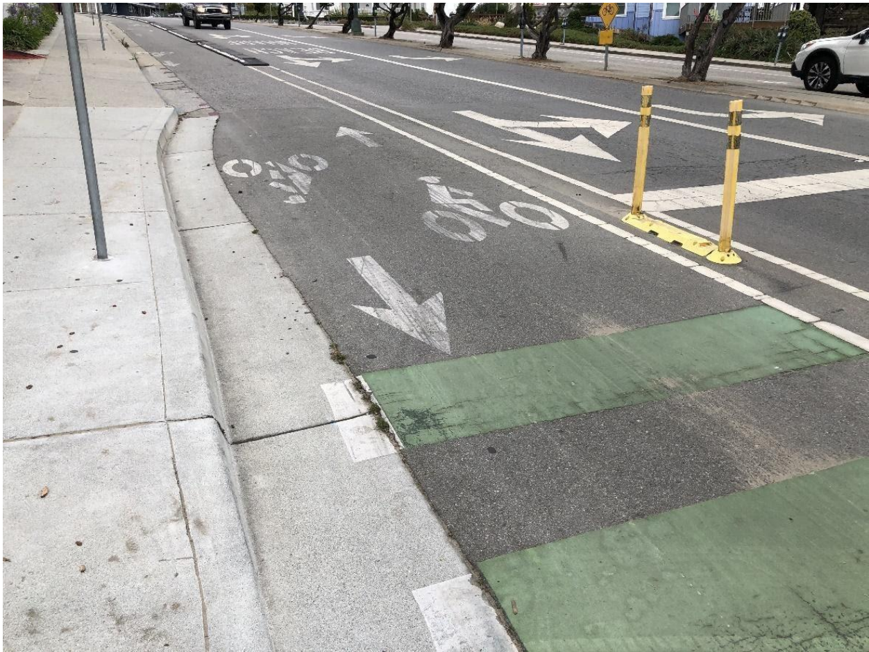
Figure 7-14. Two-way cycle track with adjacent traffic and sidewalk.
