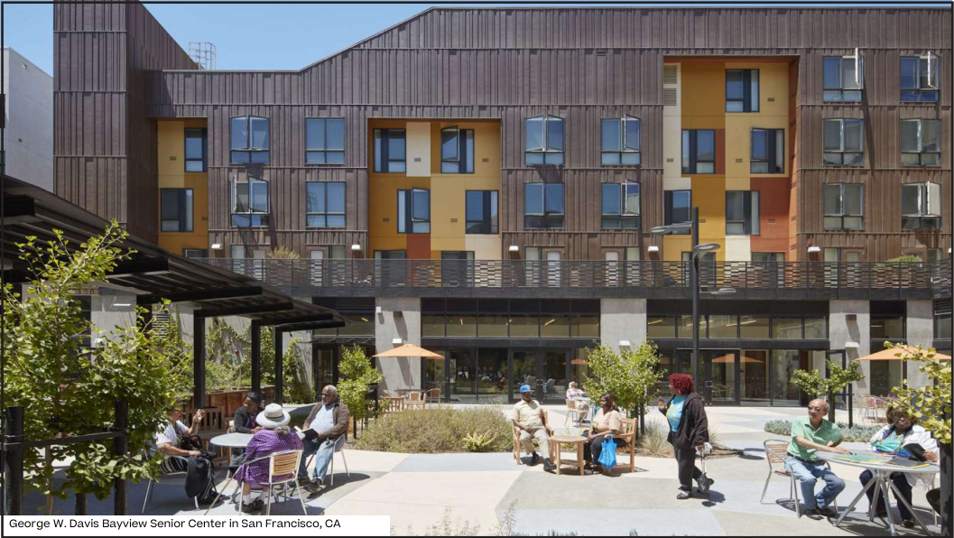
George W. Davis Bayview Senior Center in San Francisco, CA
