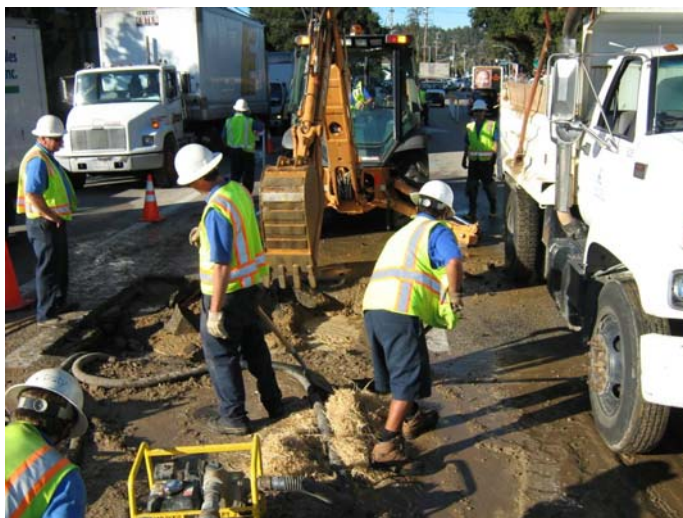
Water distribution crews working on system leak repair
