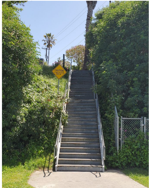
Cliff Street stairs.
