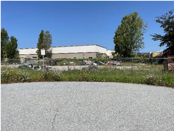
Looking north across the northern portion of the Subject Property
