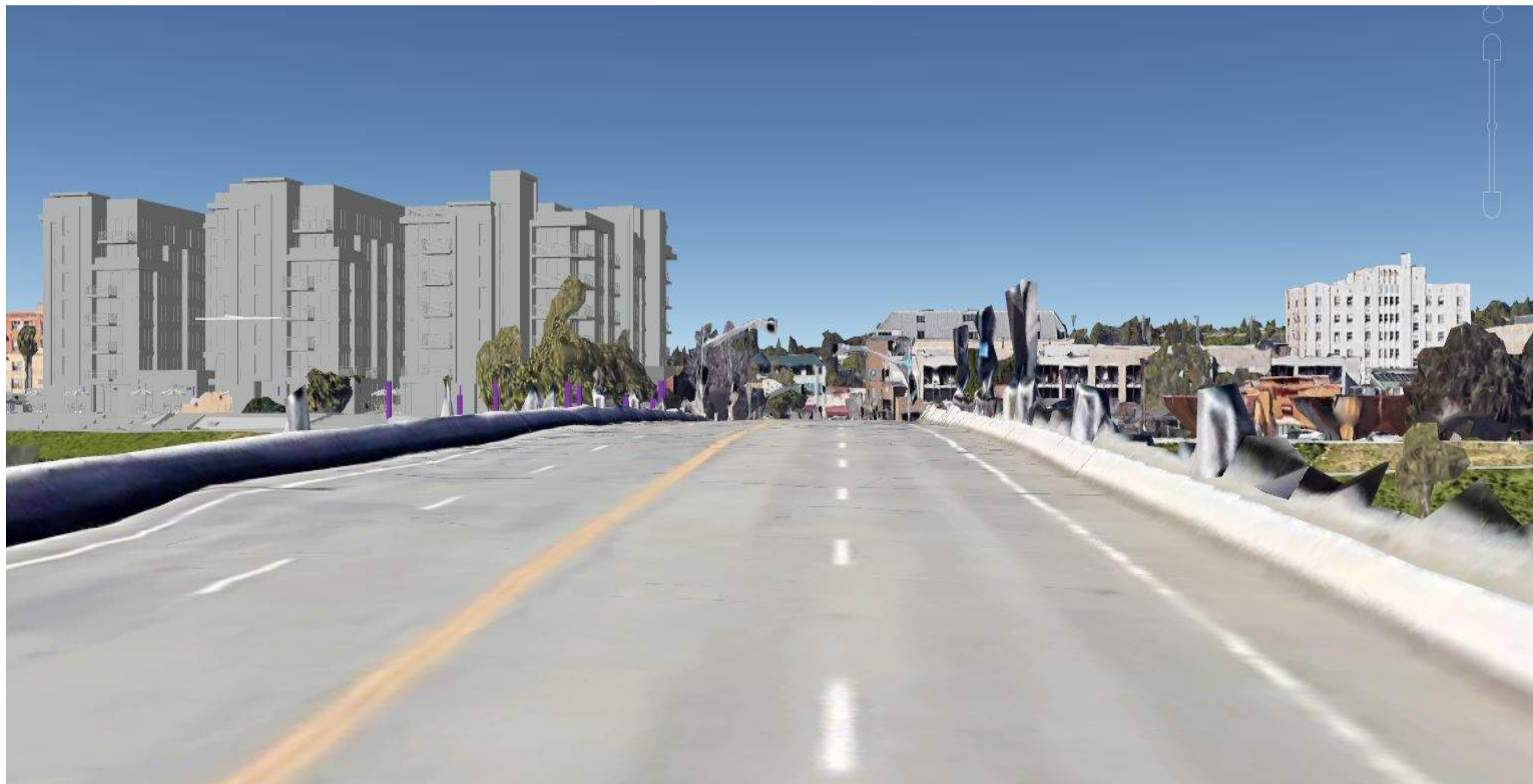
02 STREETVIEW - SOQUEL AVENUE BRIDGE 2
