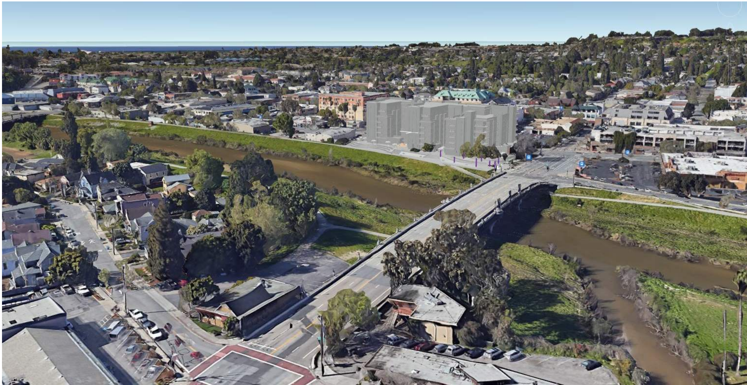
01 AERIAL - SOQUEL AVENUE BRIDGE
