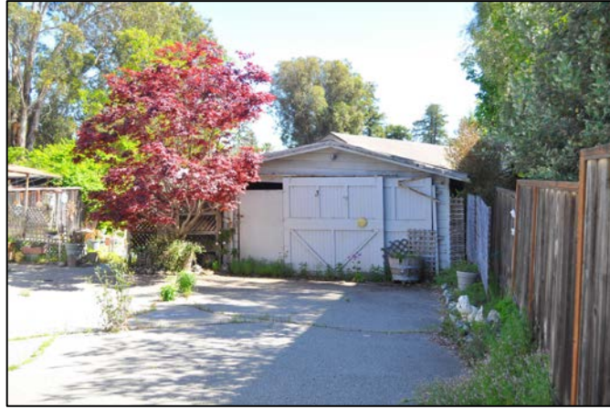
Figure 6. View of circa-1940s detached garage.
