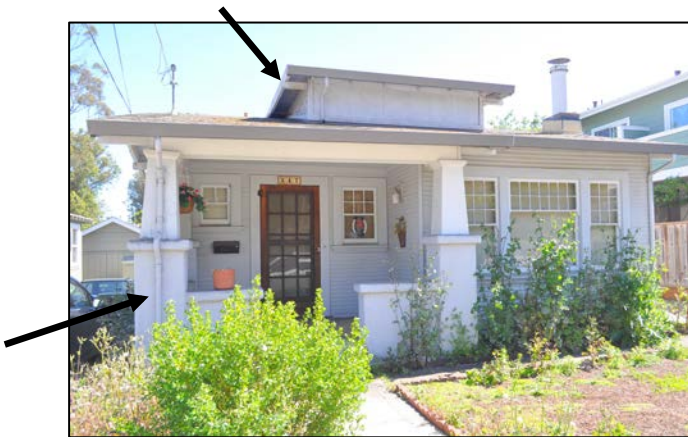
Figures 4 and 5. Left image details the front elevation, showing infilled dormer and the front porch modified with a newer concrete slab, and poorly applied stucco cladding to the original porch column bases and rails (arrows). Right image details the rear elevation, with awnings and a small rear addition.
