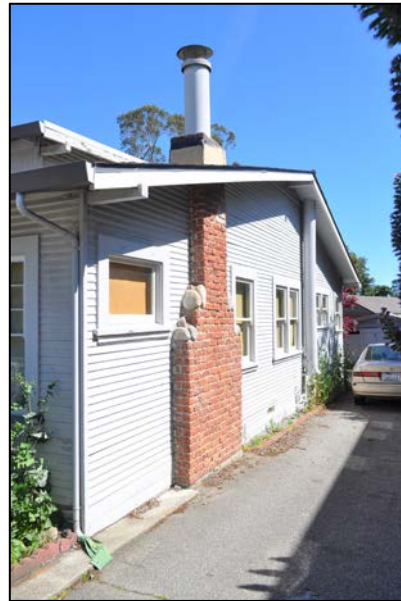
Figures 2 and 3. Left image shows the front elevation. Right image details the right side elevation with replaced fixed sash and the chimney removed at the roofline, with a metal chimney stack installed.
