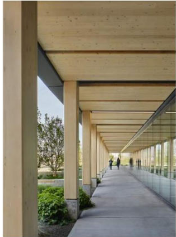
4. EXPOSED MASS TIMBER COLUMNS
