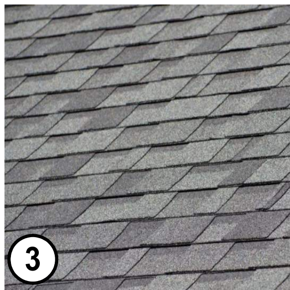
COMPOSITE SHINGLE ROOF
