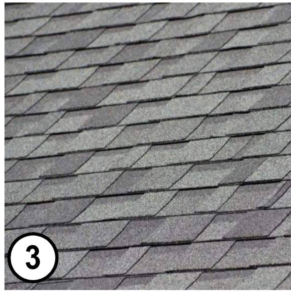
3 COMPOSITE SHINGLE ROOF
