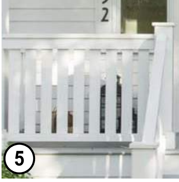
5 PAINTED DECK RAILINGS
