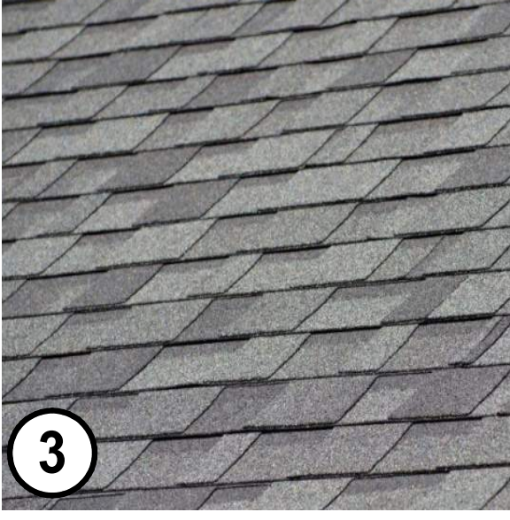
3 COMPOSITE SHINGLE ROOF
