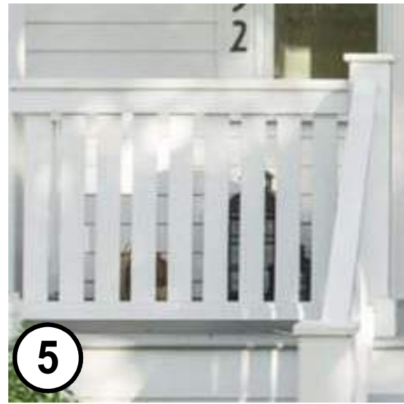
PAINTED DECK RAILINGS
