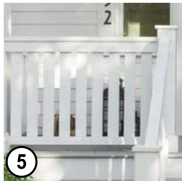
PAINTED DECK RAILINGS
