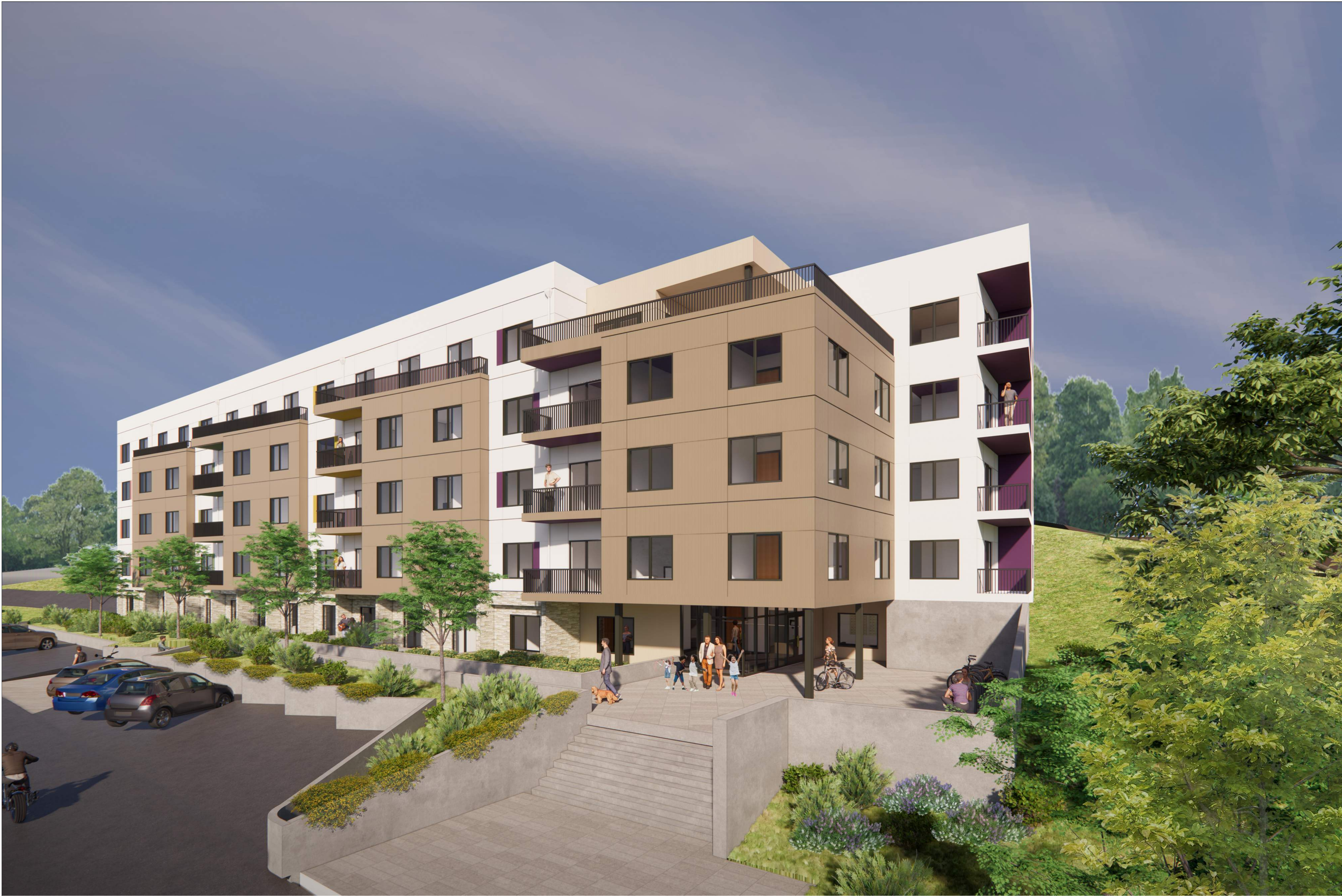
VIEW FROM SOUTH-EAST: BUILDING ENTRY
