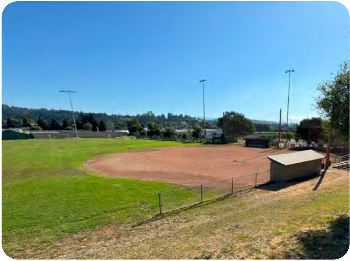
Outdated Infrastructure at Sport Fields
