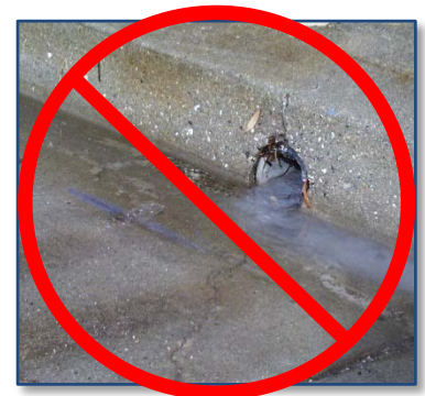
Figure 8: Do not let paint, paint thinner, or water containing either flow to the gutter or storm drain system
