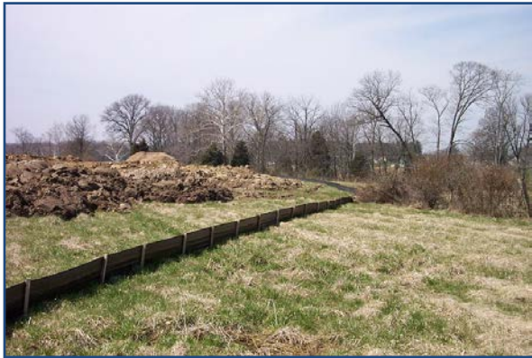
Figure 4: Perimeter silt fence
