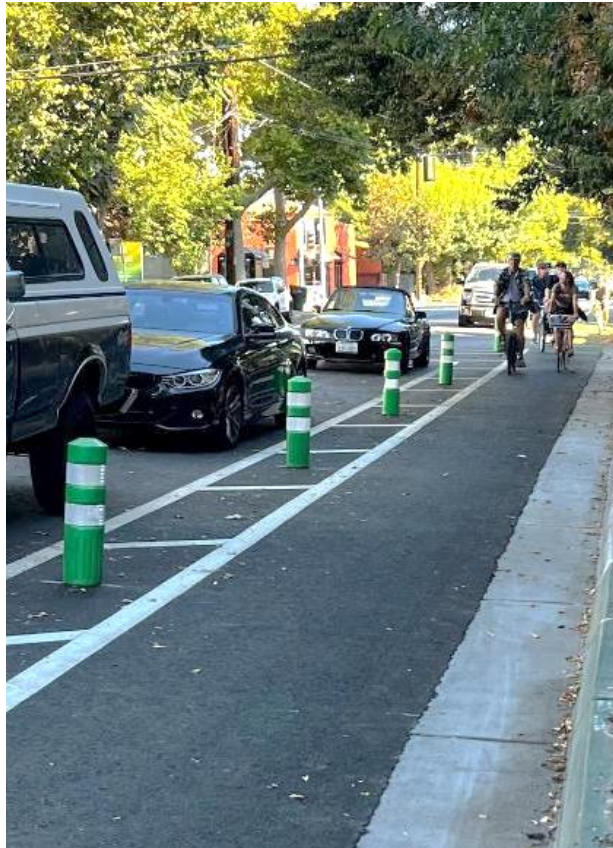
Figure 26: Bicyclists use a bollard-separated bike lane.
