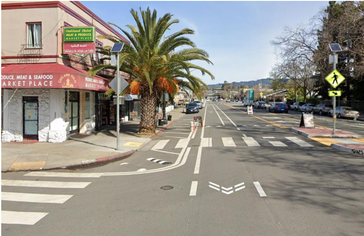
Figure 8: Slow turn wedge on an arterial in Oakland, CA
