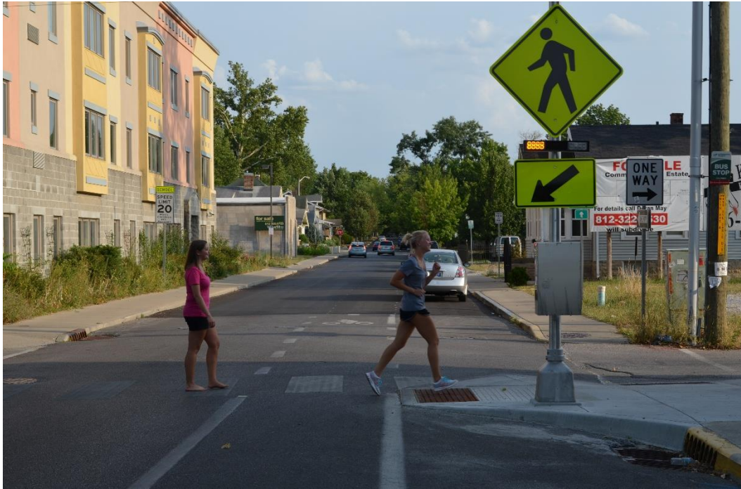
Figure 3: Rectangular rapid flashing beacon
