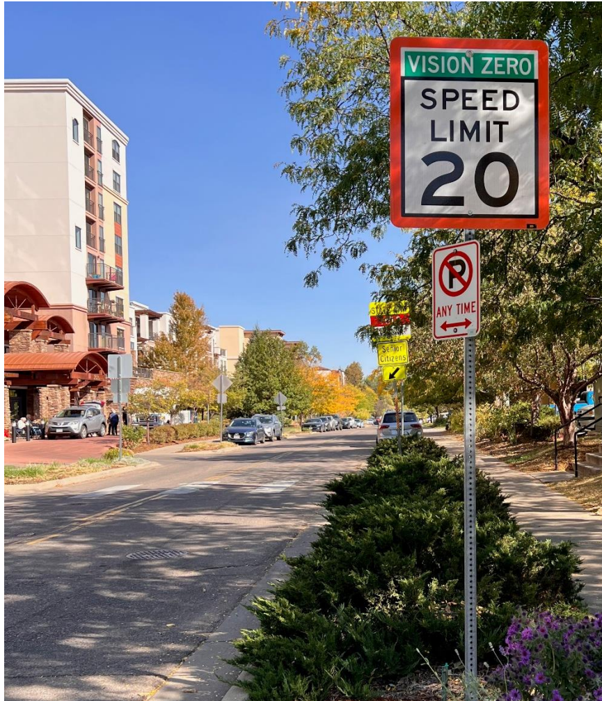
Figure 16: Reduced speed limit in Boulder paired with curb extensions at a midblock crossing
