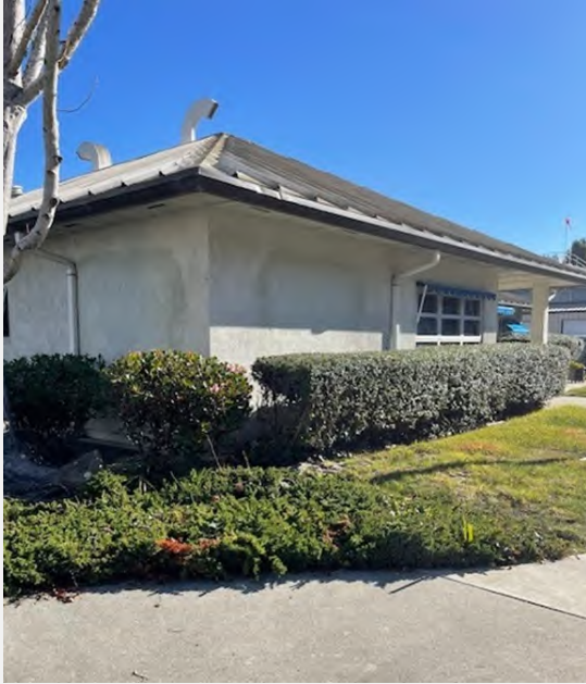
Image 005. Primary Sedimentation Structure, view north.
