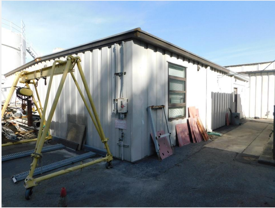
Exhibit 21. View of the Metering and Switch Unit structure, view looking north (DSCN_0148).
