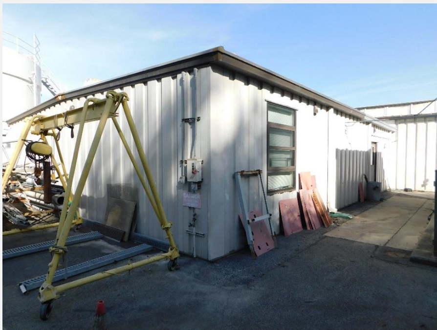
Photograph 20. View of the Metering and Switch Unit structure, view looking north (DSCN_0148).
