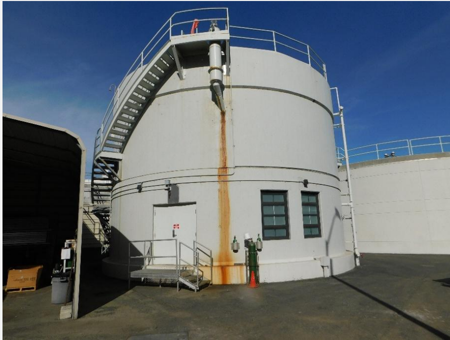
Exhibit 4. Water Tank, view looking northwest (IMG_11639).
