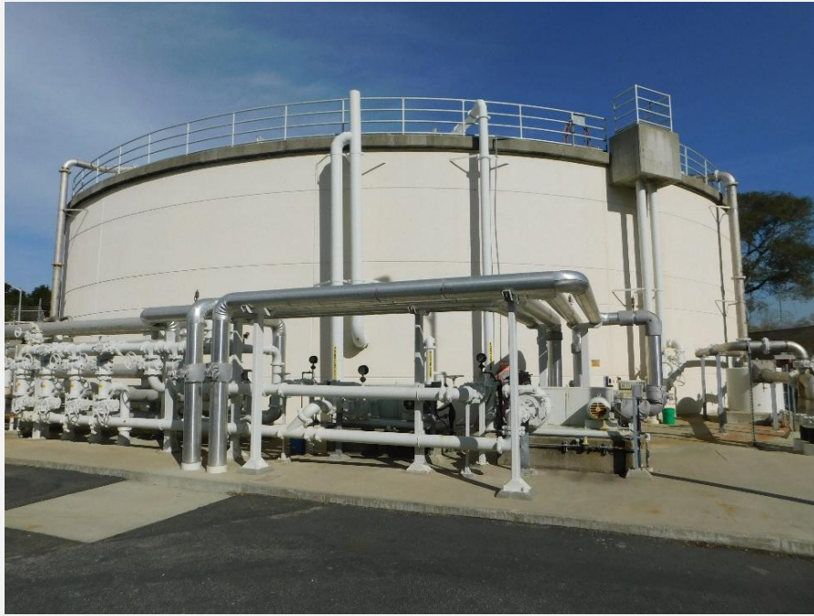
Exhibit 12. View of Digester 4, view looking southwest (DSCN_0198).
