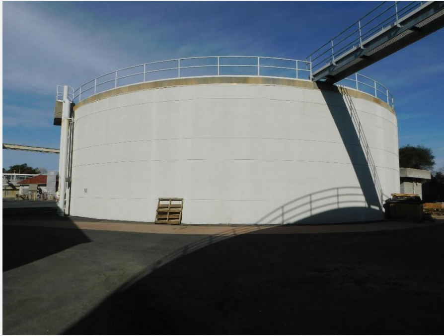
Exhibit 10. View of Primary Digester 1, view looking northwest (DSCN_0182).
