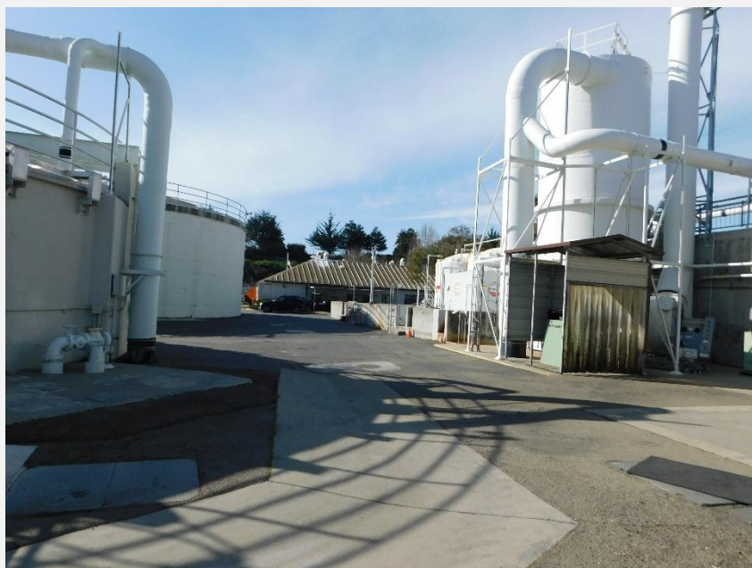
Exhibit 1. Overview of the Santa Cruz WWTF, view looking south (DSCN_0175).
