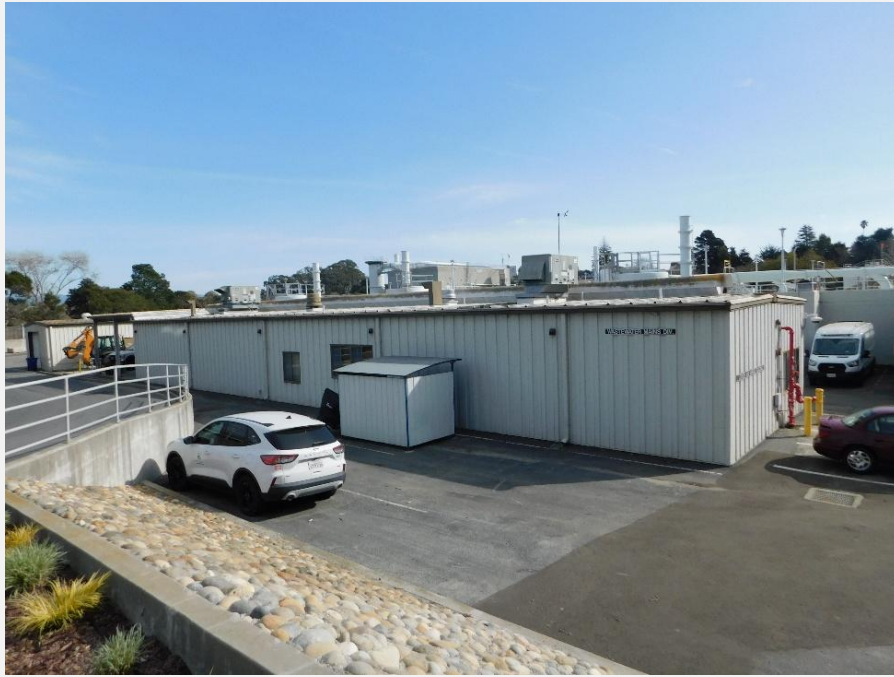
Exhibit 20. View of the Locker and Garage Building, view looking southeast (DSCN_0228).
