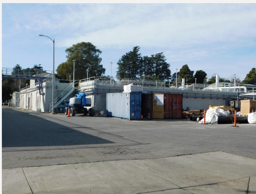
Photograph 5. Primary Sedimentation Structure, view looking southwest (DSCN_0210).
