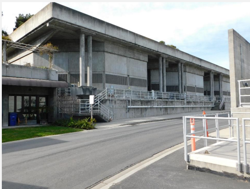
Photograph 21. View of Trickling Filters 1–6 structure, view looking west (DSCN_0239).
