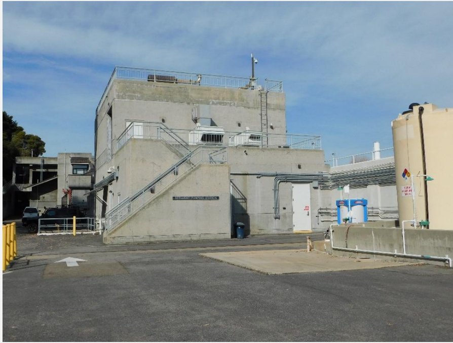
Exhibit 18. View of the Effluent Pumping Station, view looking northwest (DSCN_0218).
