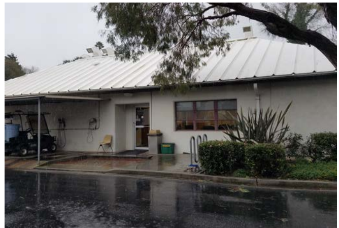
Process Control/Administration: north façade, looking south.
