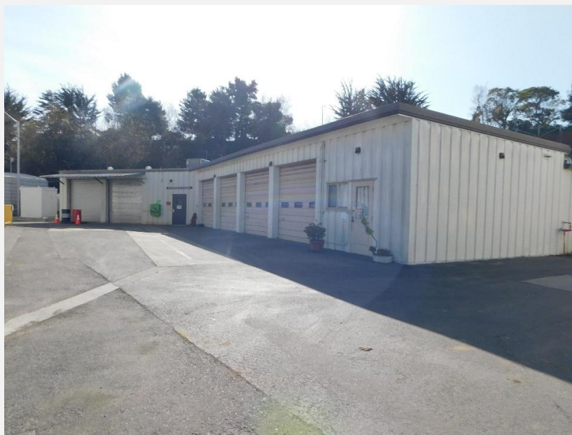
Photograph 8. View of Maintenance Building, view looking southeast (DSCN_0139).
