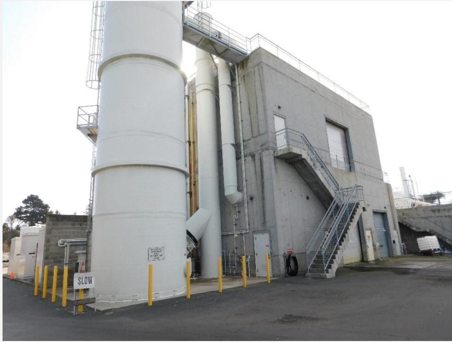
Exhibit 16. View of the Solids Dewatering Building, view looking south (DSCN_0206).
