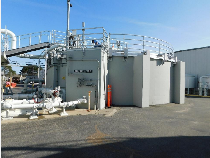
Exhibit 11. View of Thickener 2, view looking north (DSCN_0165).
