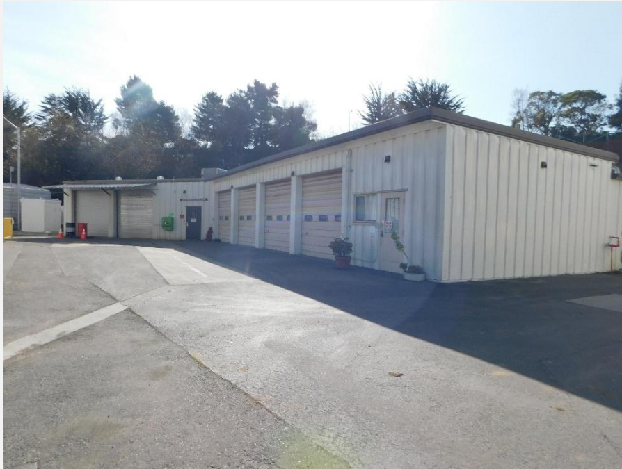
Exhibit 9. View of Maintenance Building, view looking southeast (DSCN_0139).
