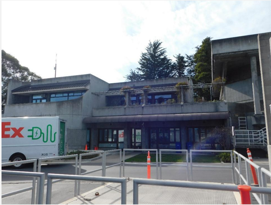
Exhibit 26. View of the (Secondary) Administration Building, view looking southwest (DSCN_0238).
