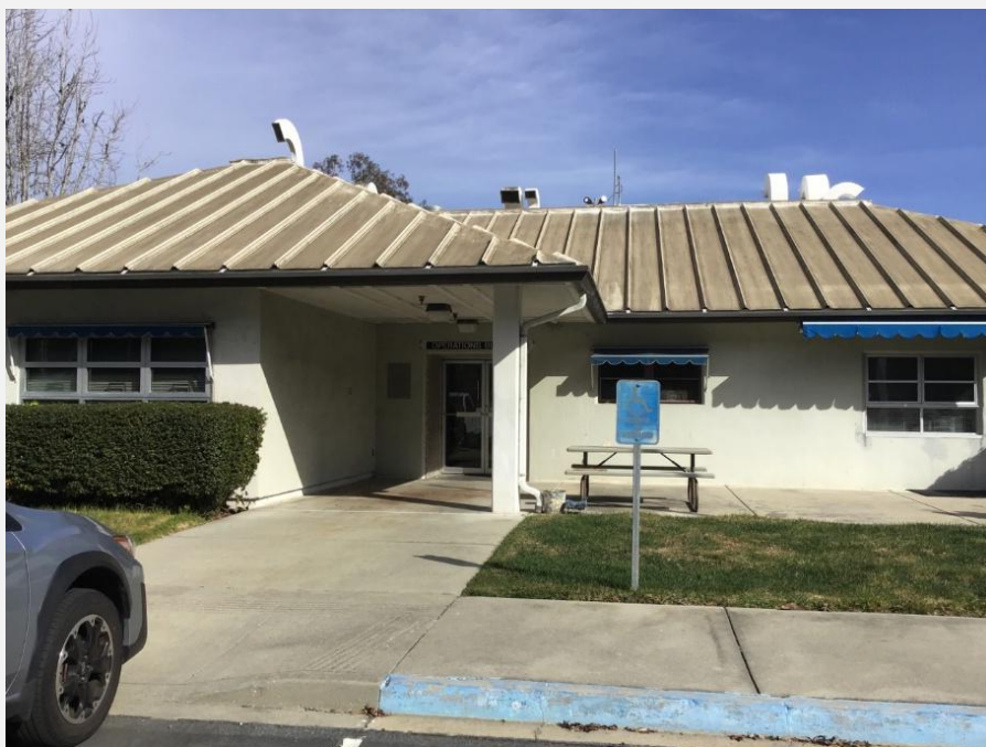
Exhibit 5. Process Control/Administration Building, view looking northeast (IMG_11637).
