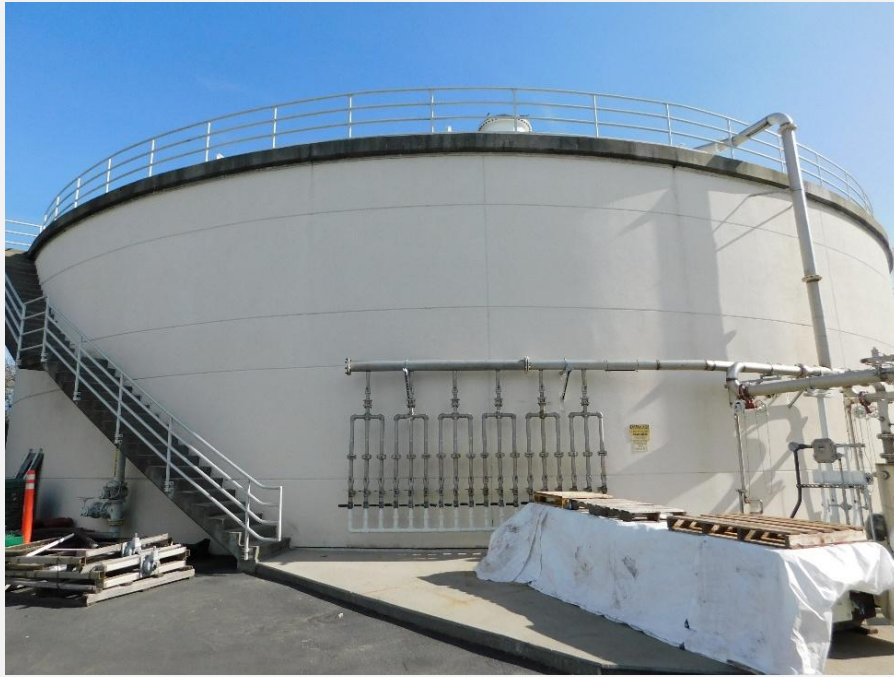
Exhibit 14. View of Digester 5, view looking east (DSCN_0197).
