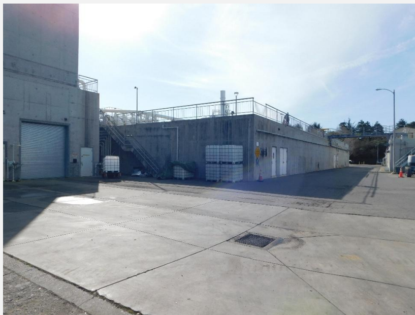
Photograph 16. View of the Preaeration Grit Structure, view looking south (DSCN_0207).
