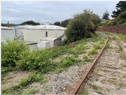
Photo Number 021. Overview of Project from SPRR, view east.
