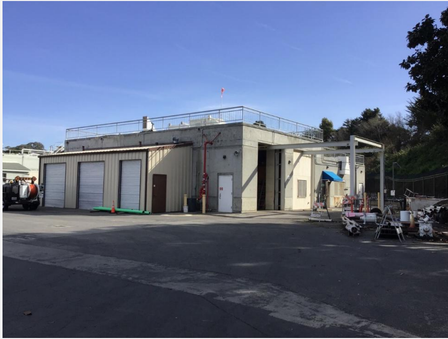
Exhibit 13. View of Electrical Building, view looking east (IMG_11638).
