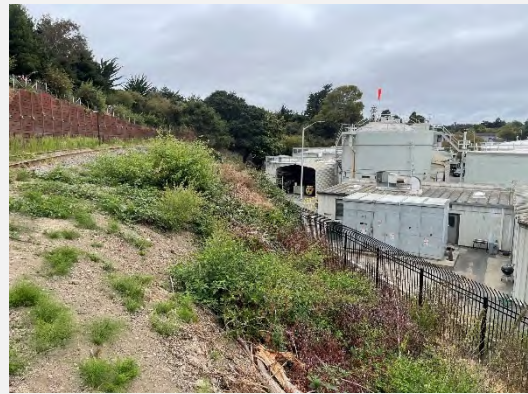
Photo Number 022. Overview of Project, view west.
