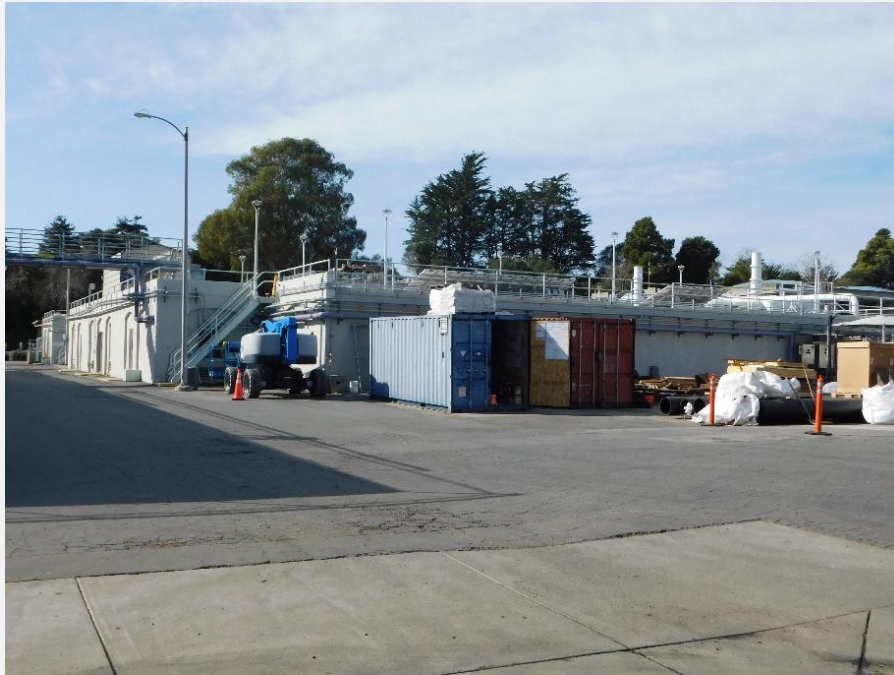
Exhibit 6. Primary Sedimentation Structure, view looking southwest (DSCN_0210).
