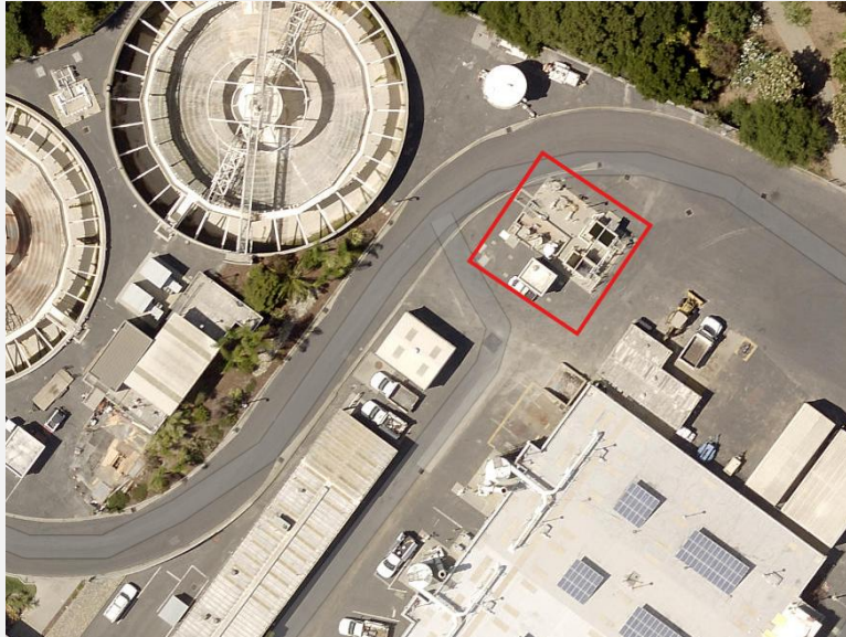
Exhibit 25. Aerial view of the Effluent Filtration structure, outlined in red (source: Esri World Imagery 2025, modified by Dudek).
