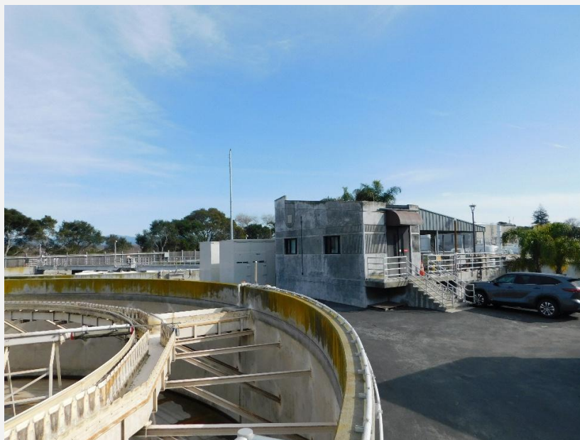
Photograph 26. View of the UV Disinfection Building, view looking northeast (DSCN_0235).
