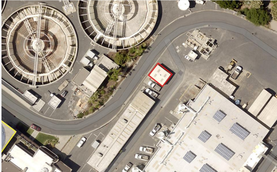
Exhibit 19. Aerial view of the UV Filtration structure, outlined in red (source: Esri World Imagery 2025, modified by Dudek).
