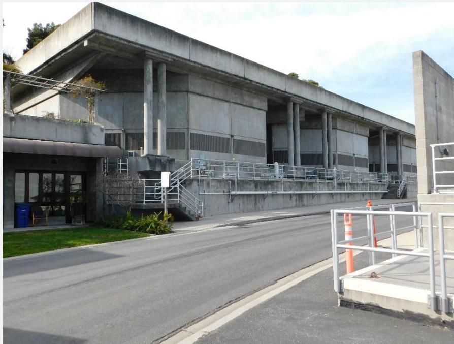
Exhibit 22. View of Trickling Filters 1–6 structure, view looking west (DSCN_0239).
