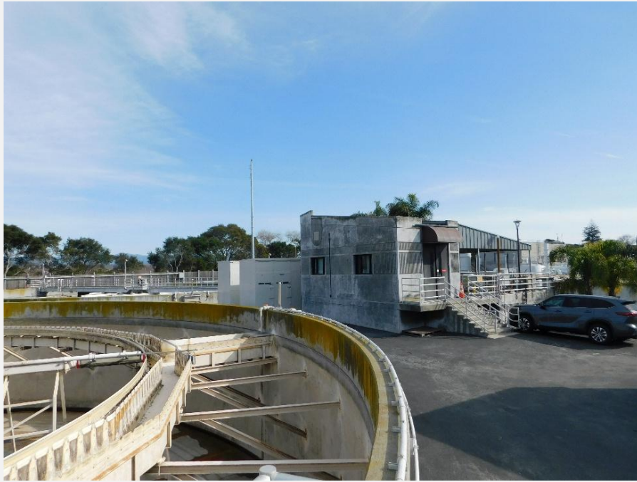
Exhibit 27. View of the UV Disinfection Building, view looking northeast (DSCN_0235).
