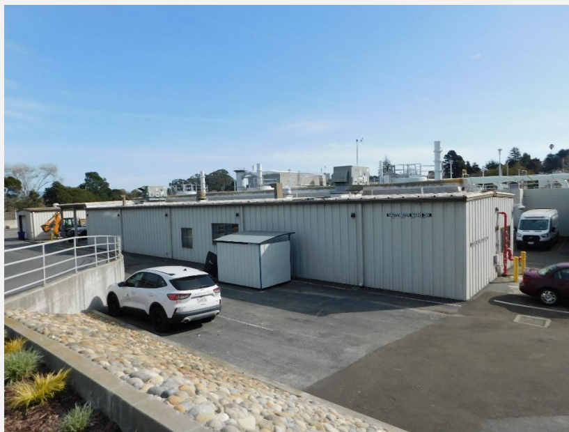
Photograph 19. View of the Locker and Garage Building, view looking southeast (DSCN_0228).
