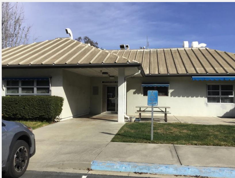
Photograph 4. Process Control/Administration Building, view looking northeast (IMG_11637).
