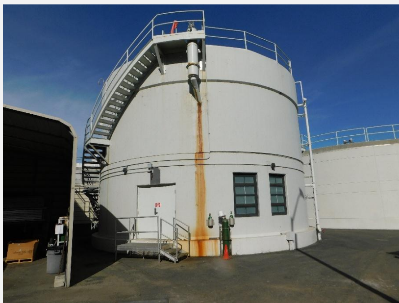
Photograph 3. Water Tank, view looking northwest (IMG_11639).
