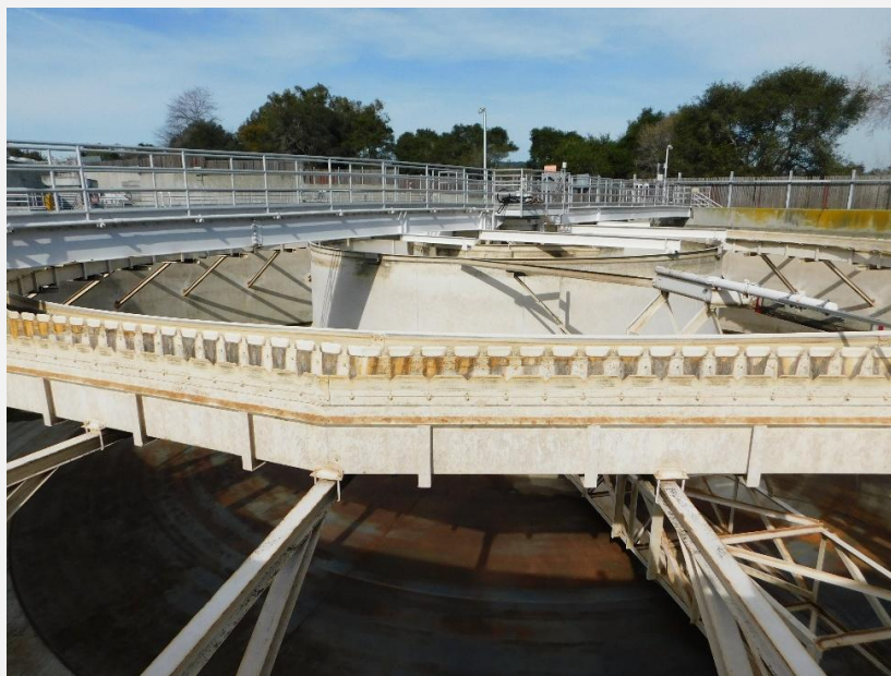
Photograph 22. View of a Clarifier Structure, view looking north (DSCN_0230).
