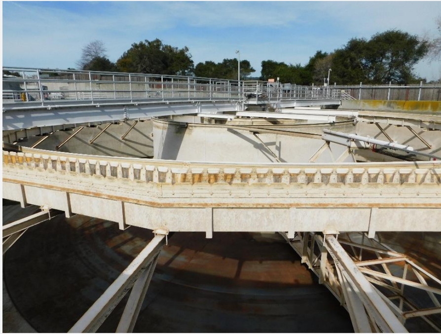
Exhibit 23. View of a Clarifier Structure, view looking north (DSCN_0230).
