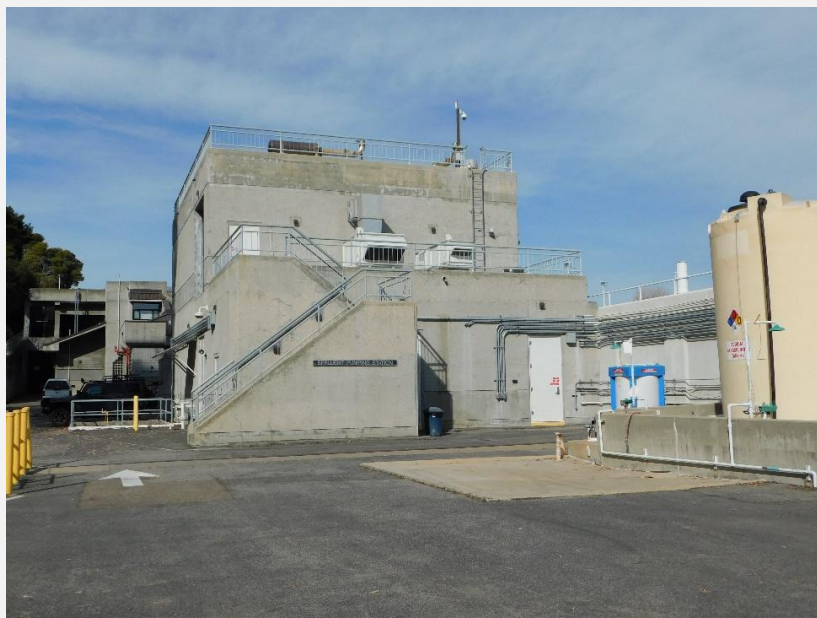
Photograph 17. View of the Effluent Plumping Station, view looking northwest (DSCN_0218).
