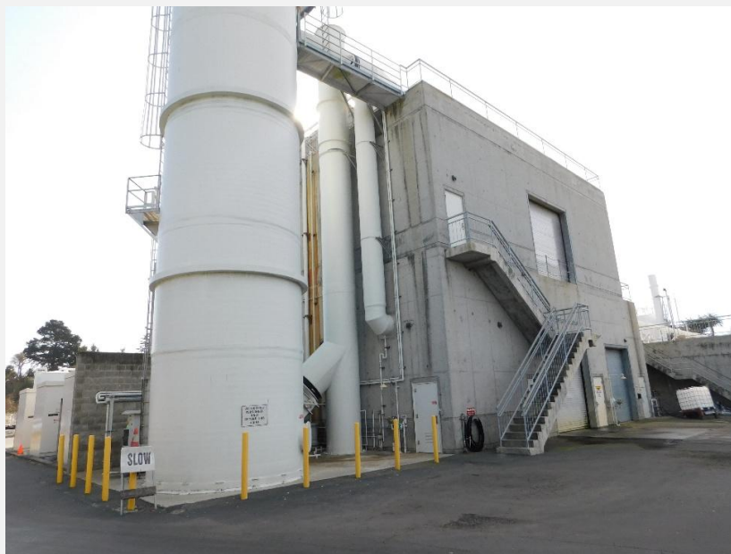
Photograph 15. View of the Solids Dewatering Building, view looking south (DSCN_0206).
