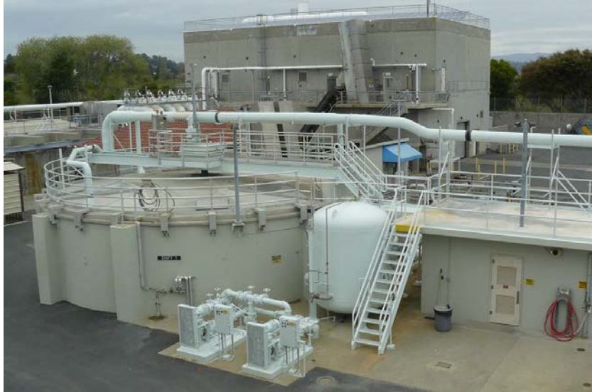
DAFT 1: south façade, looking north.
