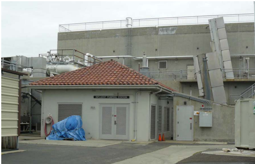
Influent Pump Station: south façade, looking north.
