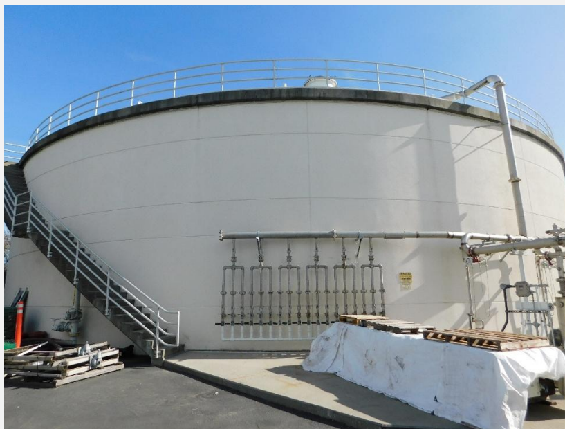
Photograph 13. View of Digester 5, view looking east (DSCN_0197).
