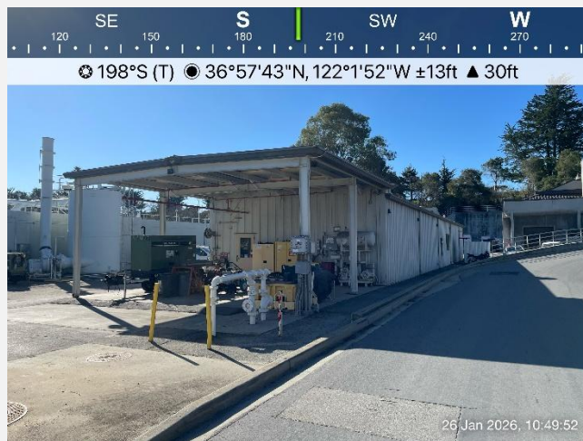
Photo 9. The building locker and garage, which will be modified to accommodate staff displaced by demolition of the maintenance building.
