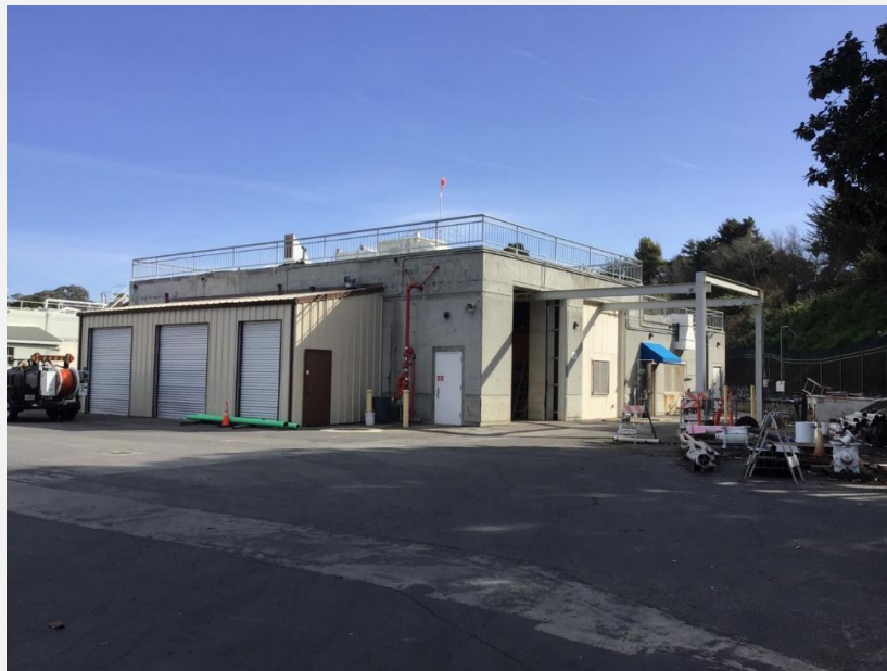
Photograph 12. View of Electrical Building, view looking east (IMG_11638).
