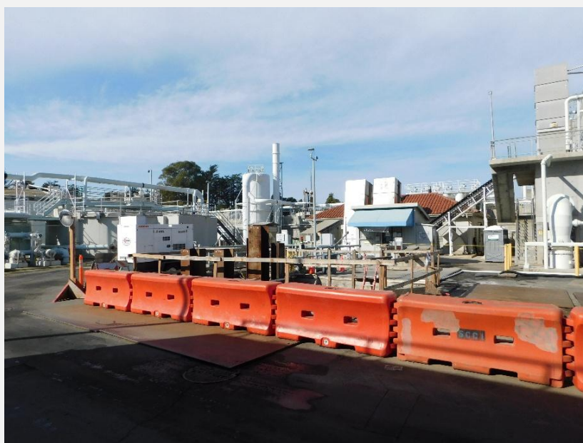
Photograph 7. Influent Pump Station, view looking west (DSCN_0190).
