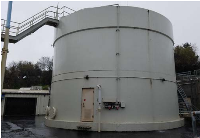
Water Tank: north façade, looking southeast.
