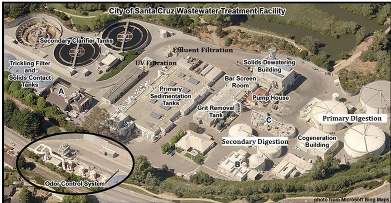
Figure 6-8: City of Santa Cruz Wastewater Treatment Facility
