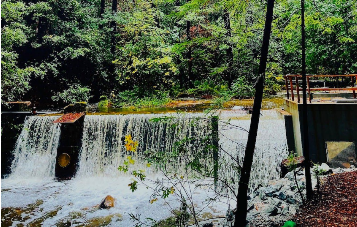
Figure 6-3: Laguna Creek Diversion Dam
