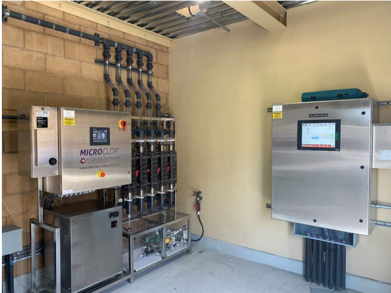
City of Santa Ana Walnut Well OSHG Installation
