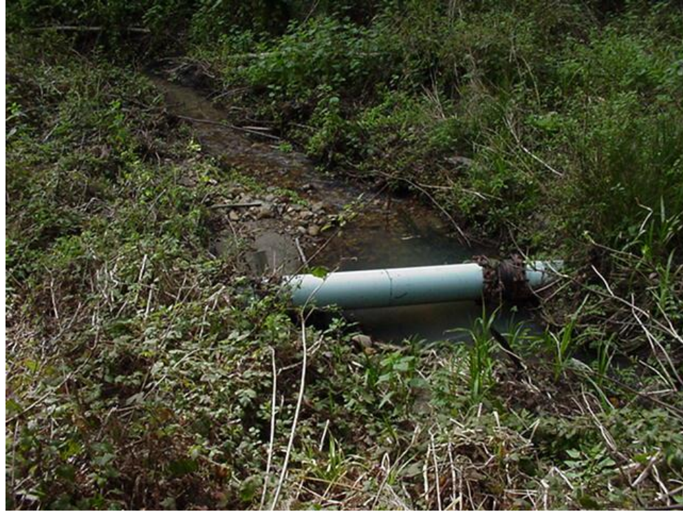
Photo A7 - Liddell Reach and LID-Alt. - Pipeline Crosses Yellow Bank Creek Crossing (LID-02) Downstream of Road and Culvert (p.d. 6,400 feet)
