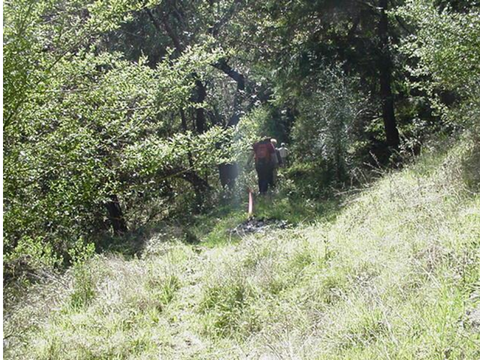
Photo A1 - Liddell Reach - ROW on Slope - Pipeline to the Left Downstream from Liddell Springs (p.d. < 500 feet)
