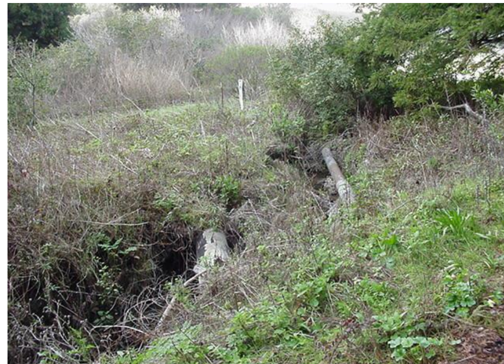
Photo A26 - Laguna/Liddell Reach - Pipeline Ditch Crossing (p.d. 3,200 feet)
