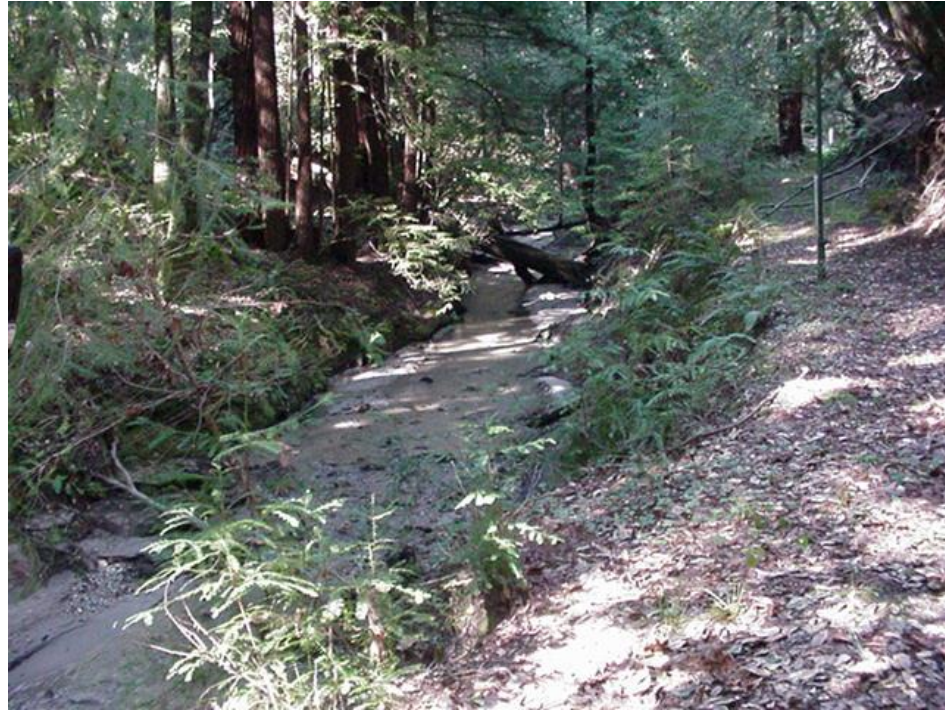
Photo A31 - Majors Reach - Pipeline to the Right of Majors Creek, Adjacent to Riparian Corridor (p.d. 500 to 1,500 feet) (Upstream View)
