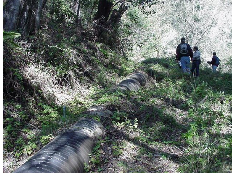
Photo A2 - Liddell Reach - Pipeline to the Left of the Drainage Pipe Along the Ridgeline (p.d. 1,000 feet)
