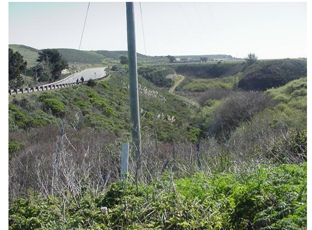
Photo A44 - NCP Reach and NCP Alt. - Pipeline Goes Into Ravine at NCP-04 Baldwin Creek (p.d. 10,500 feet)
