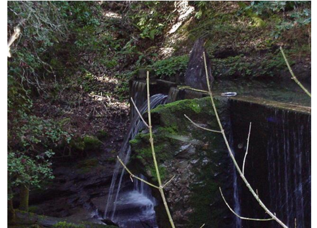
Photo A29 - Majors Creek Diversion - Eroded Western Bank
