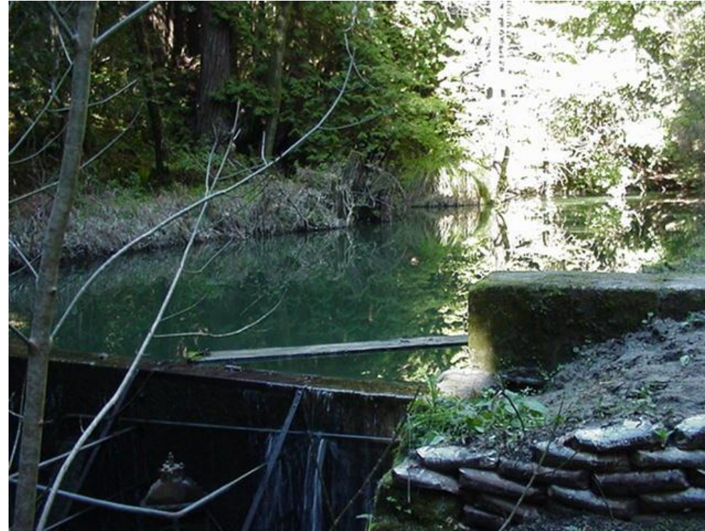
Photo A28 - Majors Creek Diversion - Looking Upstream
