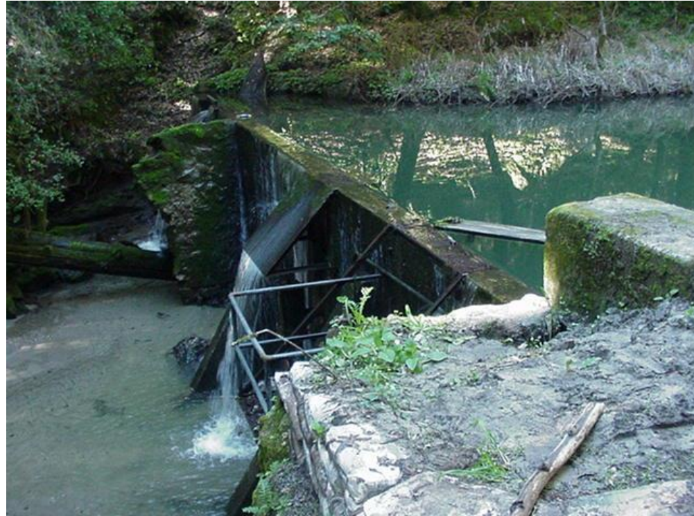
Photo A27 - Majors Creek Diversion and Impoundment
