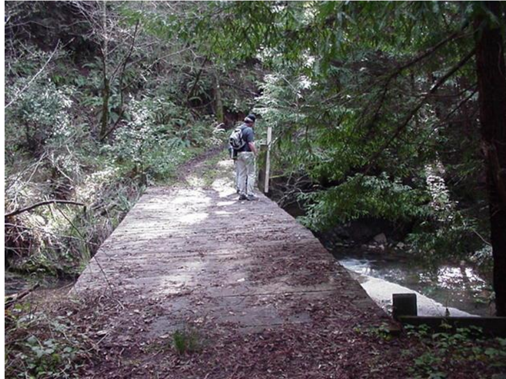
Photo A14 - Laguna Reach - Pipeline Crossing LAG-02 Stream Crossing- pipeline is Buried (p.d. 2,900 feet)
