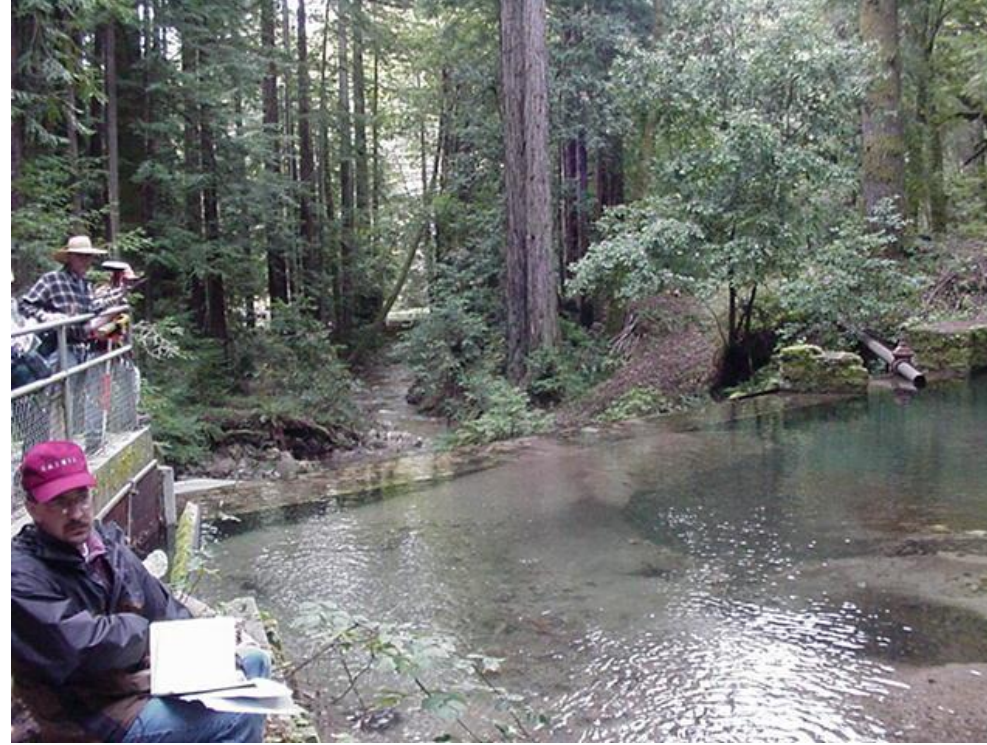
Photo A11 - Laguna Creek Diversion Intake and Impoundment
