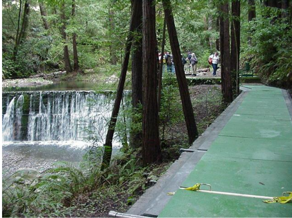
Photo A10 - Laguna Creek Diversion and Flume
