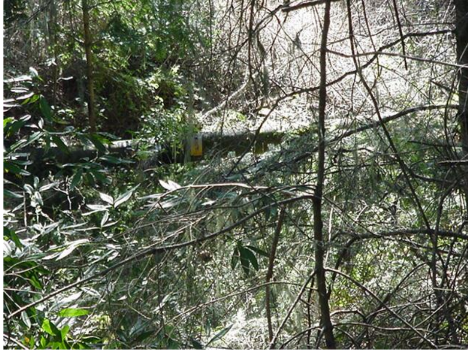
Photo A37 - Majors Reach - Leaky Pipeline Crossing Over a Ravine. Typical Conditions (p.d. 3,000 to 8,000 feet)
