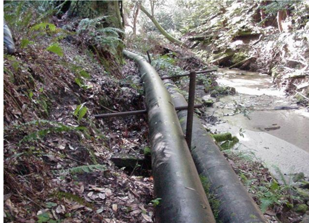
Photo A32 - Majors Reach - Pipeline to the Left of Majors Creek, Smaller Pipes Present to Support Unstable Pipeline (p.d. 500 feet)
