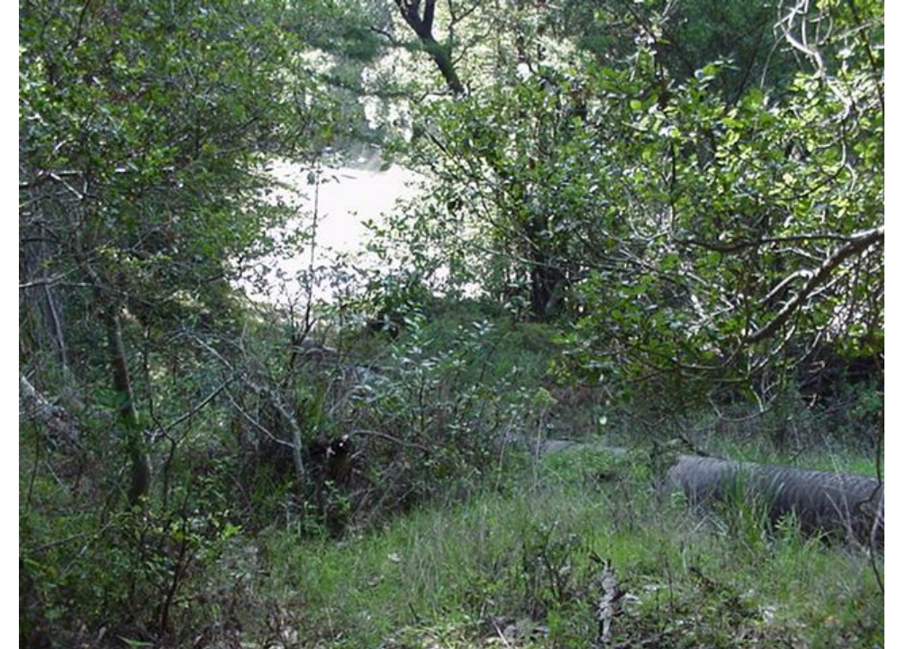
Photo A3 - Liddell Reach - Pipeline on Ridgeline Drainage Pipe to Quarry Settling Ponds (p.d. 1,300 feet)
