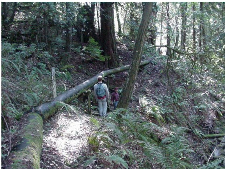
Photo A34 - Majors Reach - Pipeline Suspended on Trestles Over a Small Ravine. Typical Conditions (p.d. 2,500 to 5,000 feet).
