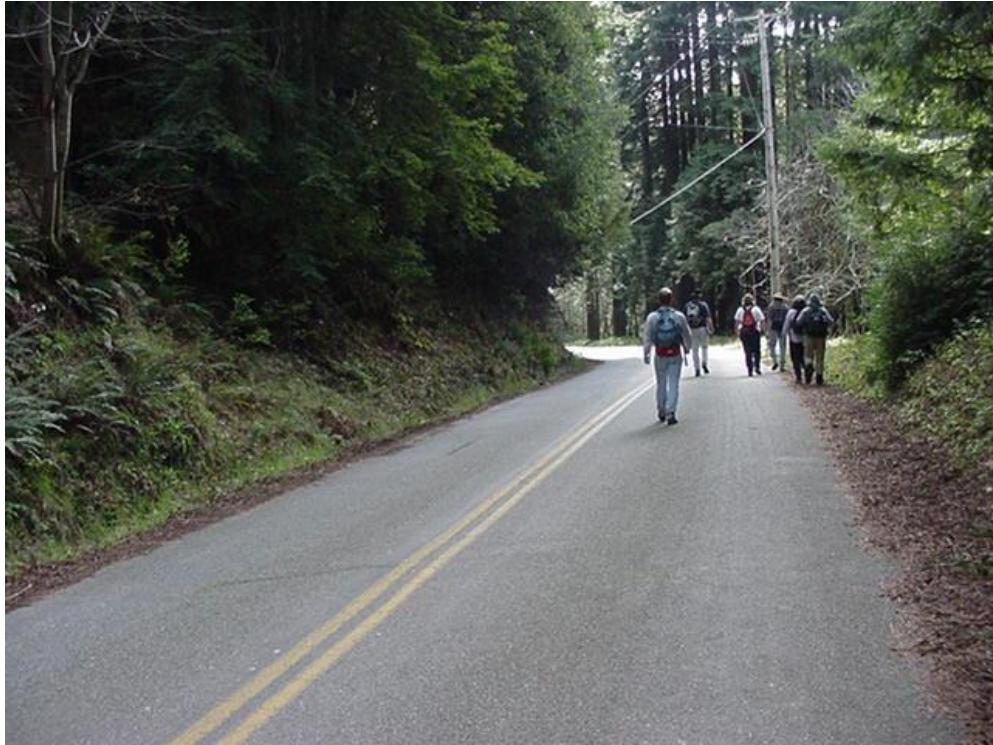
Photo A13 - Laguna Reach - Pipeline Underground Following Smith Grade Road (p.d. 0 to 1,500 feet)
