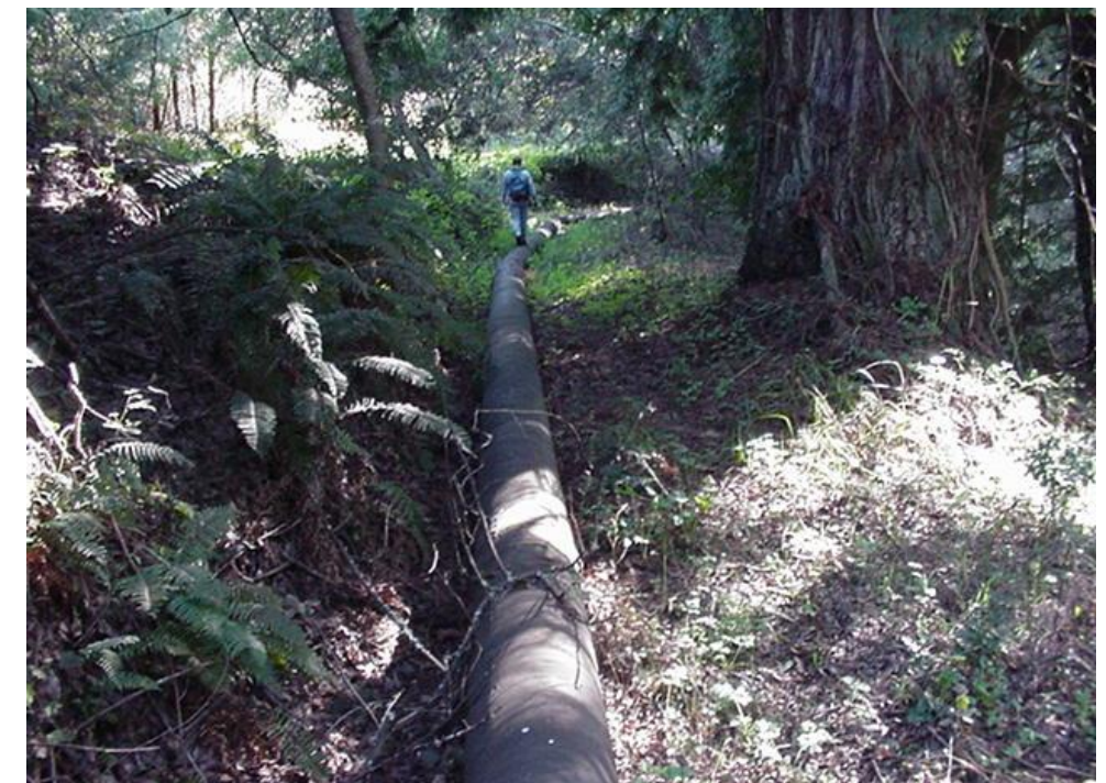
Photo A36 - Majors Reach - Following Pipeline Through Broadleaf Evergreen Forest-Road is to the Left (p.d. approximately 2,500 feet)
