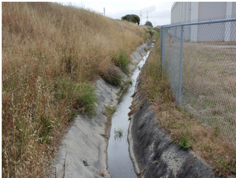
Photograph 10. Concrete stormwater drainage ditch below seasonal wetland draining to stormdrain
