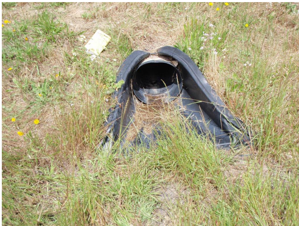
Photograph 9. Stormwater culvert draining from Arroyo Seco Creek floodplain to seasonal wetland
