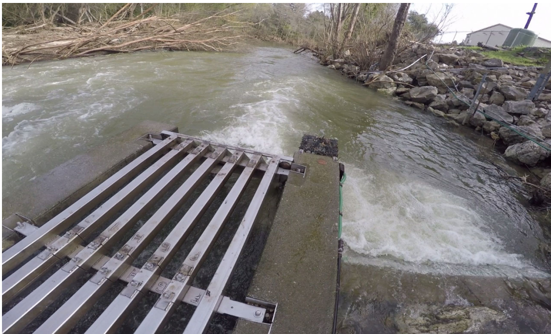
TAIT DIVERSION FACILITY – LOOKING DOWNSTREAM
