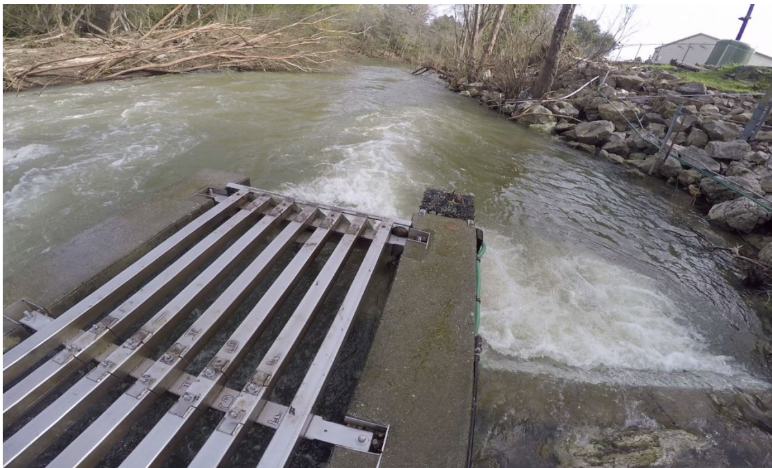
TAIT DIVERSION FACILITY – LOOKING DOWNSTREAM
