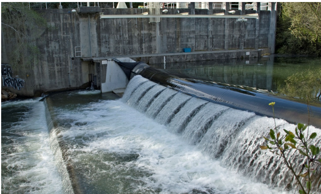
FELTON DIVERSION FACILITY
