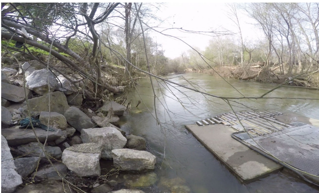
TAIT DIVERSION FACILITY- LOOKING UPSTREAM
