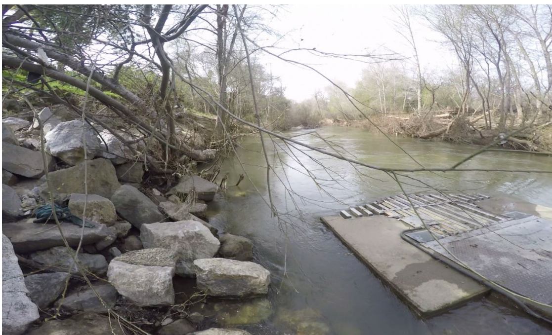
TAIT DIVERSION FACILITY- LOOKING UPSTREAM
