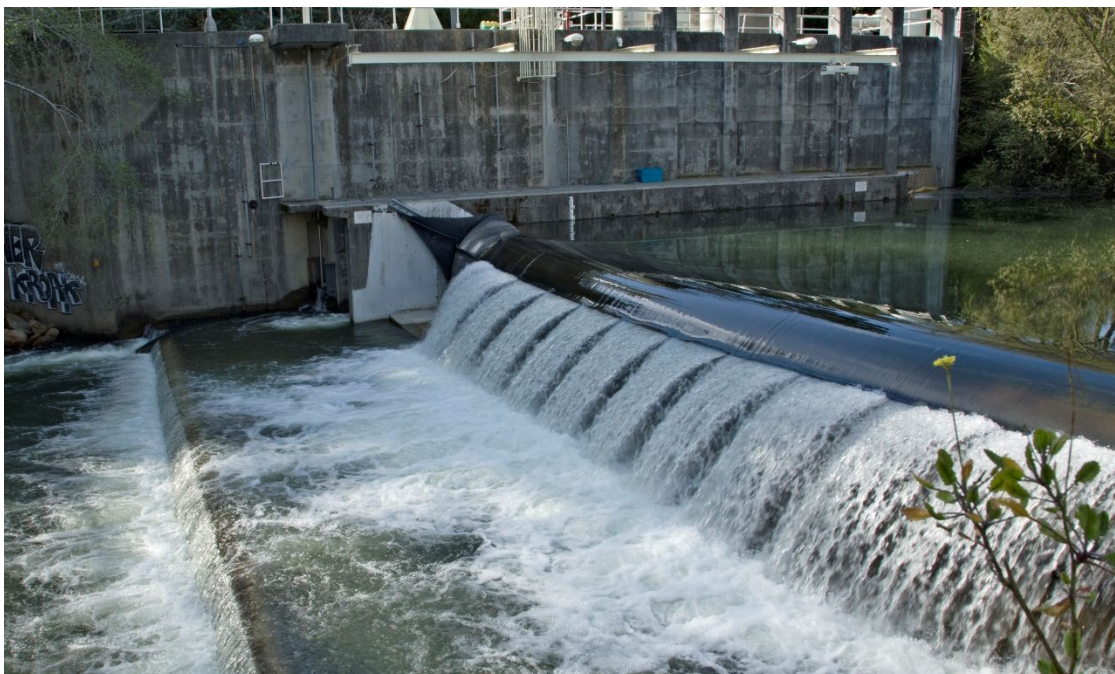
FELTON DIVERSION FACILITY
