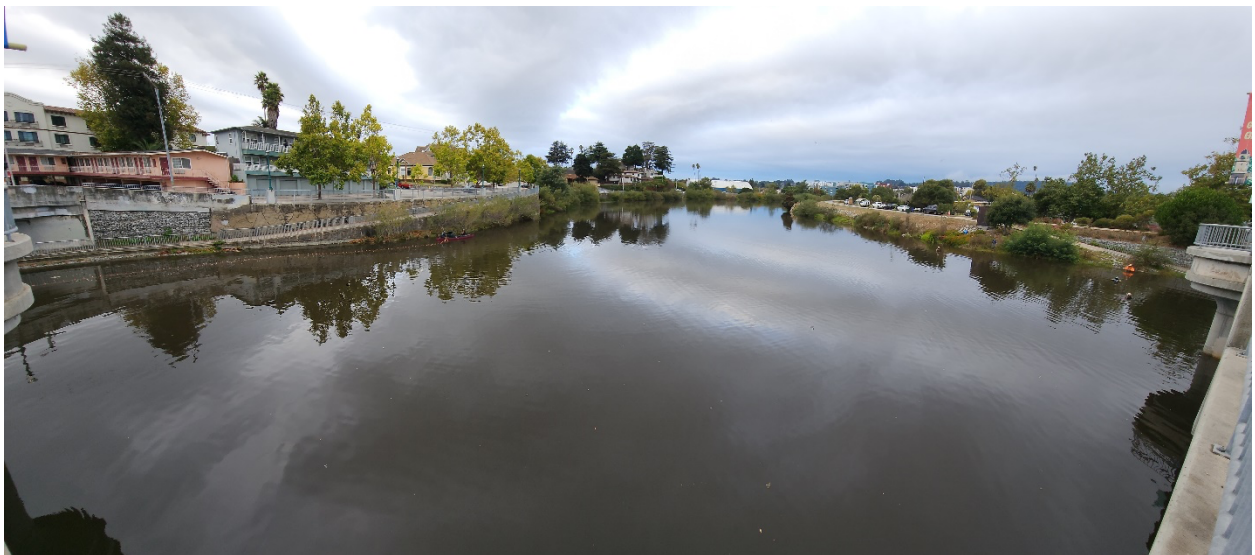
Figure 20. San Lorenzo River upstream of Riverside Bridge October 15, 2025 (pre-breach)
